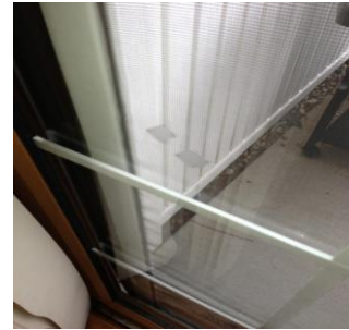
Tape on Windows/Glass
