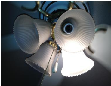
Missing/Burned Out Light Bulbs
